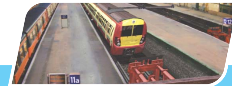
New platform created at Glasgow Central Station
