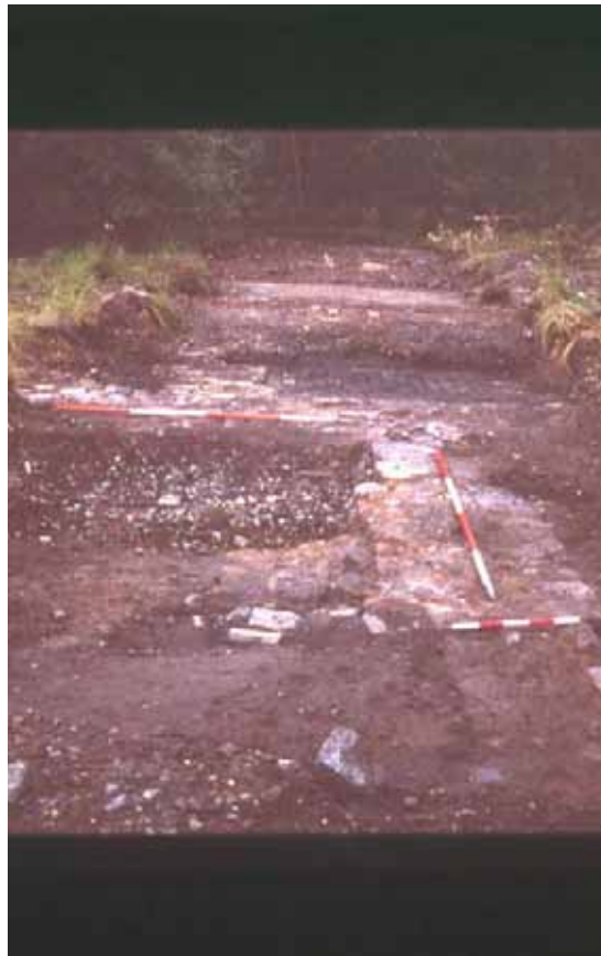
Trench 16 Various structures within northern row including stone foundations, brick floors, cement surfaces.
