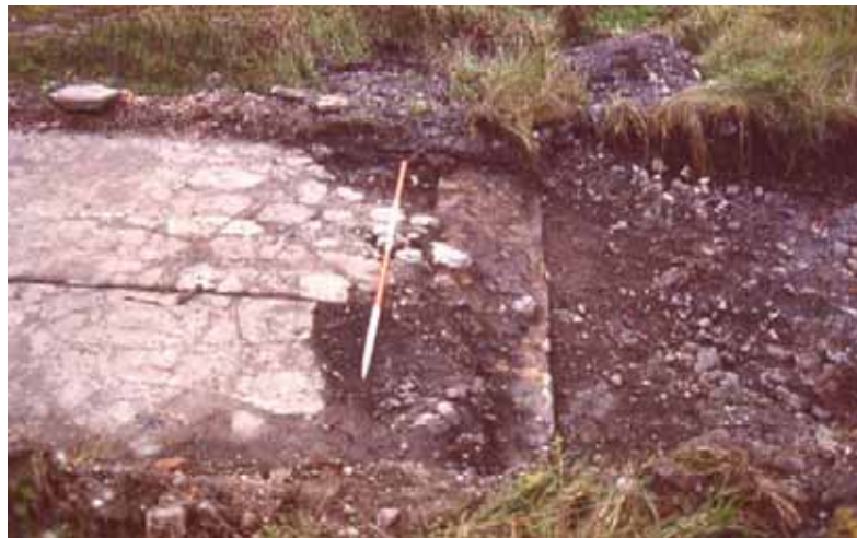
Trench 15 showing stone built foundations and cement surfaces.
