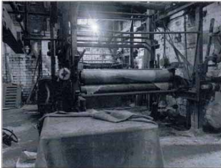
Rolling machine that coated the cloth with gas proof chemicals SCRAN ID 000-000-184-767-C
